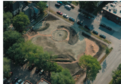
Aerial view of the park under construction.
